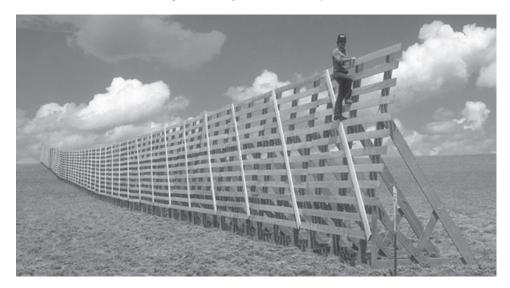
Figure 12.2 Wyoming snow fence that has been extensively tested and used to control blowing snow in Western United States (Tabler 2003, © 2003 by Ronald D. Tabler, all rights reserved. Reprinted with permission).
